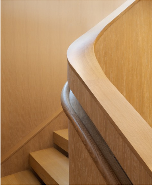
Traditional wood bending techniques achieve the carved, subtractive handrail detail
