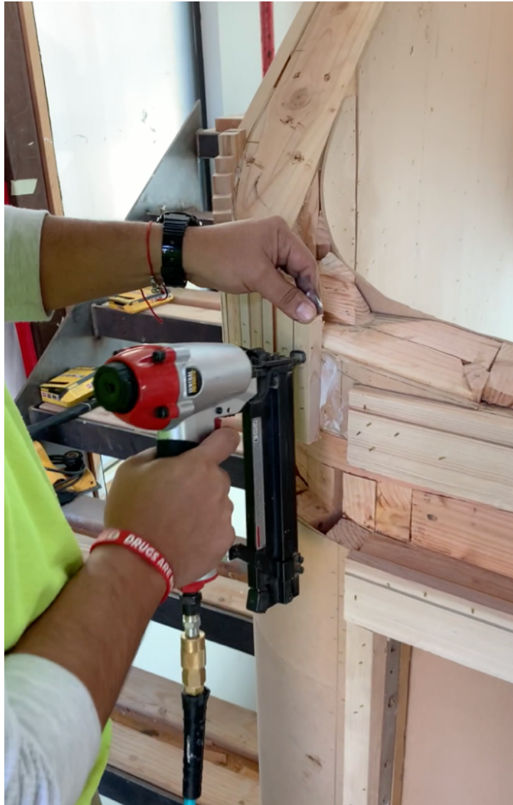
Hand-stapled wood strips provide the structure of this curved wood stair
