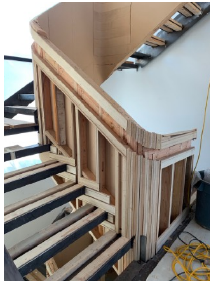
Hand-stapled wood strips provide the structure of this curved wood stair
